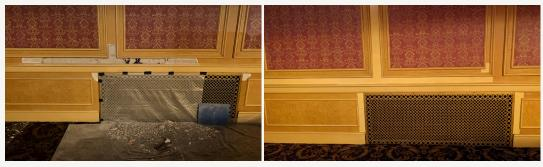
To the right is a portion of orchestra emergency exit stairs that needed similar plaster and touch up work. Much of the walls and doors in the orchestra will need similar repair and restoration.
