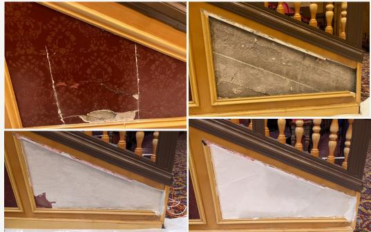
Before plaster can be layed an adhesive layer is placed down first. This is used to bind the plaster so it will adhere to the wall. That adhesive layer can be seen peaking out in the bottom left corner image before the white plaster covers it.
