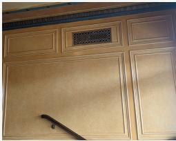
The 2nd floor men's restroom also had plaster repair work done just in time for the opening of FUNNY GIRL. Temperature fluctuations and vibrations from the moving of individuals, objects, and sound waves from the shows cause fractures and cracks to appear in the plaster due to its delicacy and sensitivity. The basement level men's restroom will need similar repairs and restoration. This has been identified as a summer project due to the estimated time and expansive repair needed.
