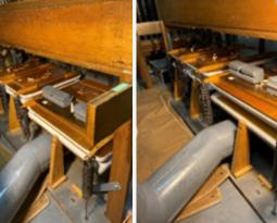
Metal windlines connect the regulators to the appropriate windchests and subsequently feed the pipes. The primary pneumatic and valve systems of the chests are the mechanical controls for determining which pipes get wind from the input at the console from the organist.
