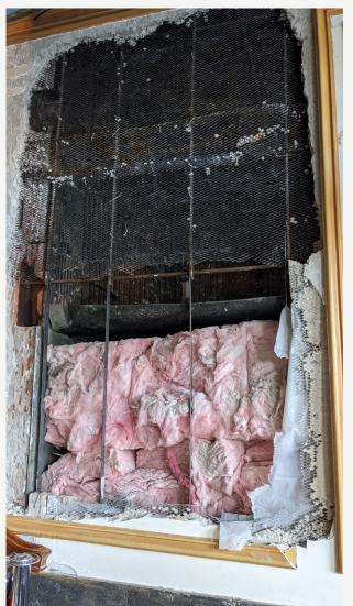
A radiator had once been located on the lower part of that wall which was approved for removal due to the high heat it produced in the infirmary.
