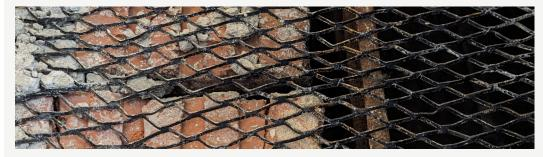
The full restoration of the wall will take at least another month to complete. This includes creating a uniform structure of restoration appropriate material across the length of the wall to reduce cracking. Then the painting of the new plaster will include the techniques of glazing, ragging, stippling, and dry brushing to match the original paint.
