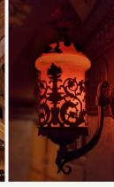
Shea's has recently applied for a \$50,000 grant for the restoration and maintainance of our dome and cylinder lights. Each fixture must be custom fabricated from mold creation to glass production, dying the material perfectly to replicate the color for when the lights are both on and off. That difference in color can be observed in the photo comparison above and below.
